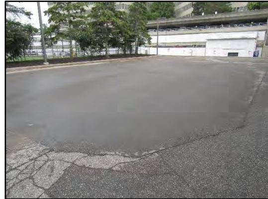
General view of a partial replacement of the asphalt pavement observed on the west portion of the site (replaced in 2019).
