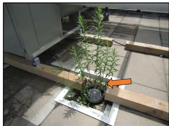
Vegetation growth observed at the roof drain location observed on the main roof area.
