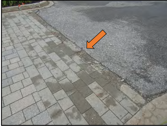
Deterioration in the pavers observed on the south portion of the site.
