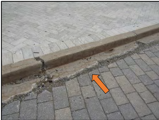
Cracking and deterioration in the concrete curb observed on the southwest portion of the site.
