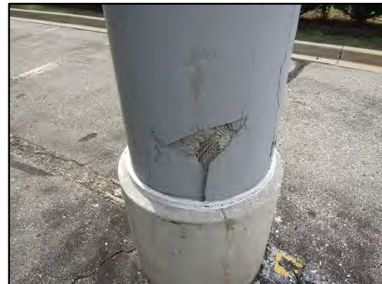
Typical impact damaged fibre cement panels observed on the ground level.
