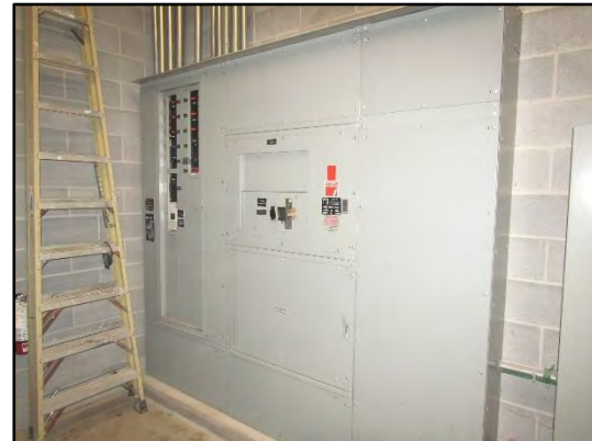
Main disconnect switchgear.
