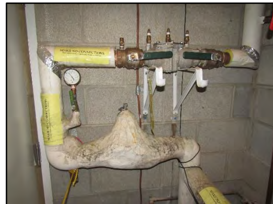
Watts 2-inch backflow preventer installed onto the main water incoming line.
