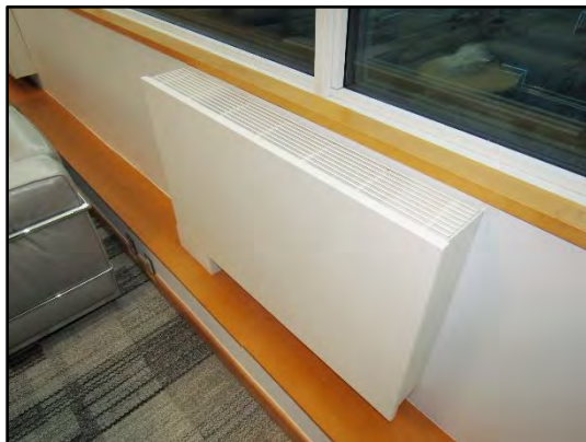
Wall mounted fan coil.
