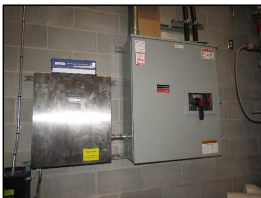
Solar photovoltaic energy system disconnect switch.
