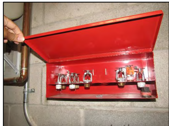
Missing installation tool and sprinkler heads observed in the sprinkler room.
