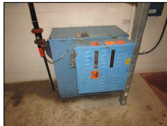
General view of the hydraulic reservoir and main elevator control panel observed in the elevation machine room.
