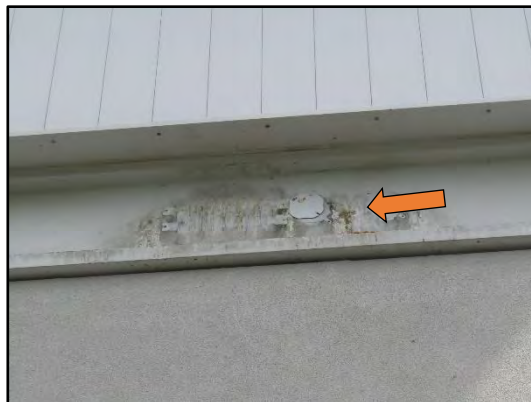
Discolouration and staining on the aluminum panel observed on the south elevation of the building.
