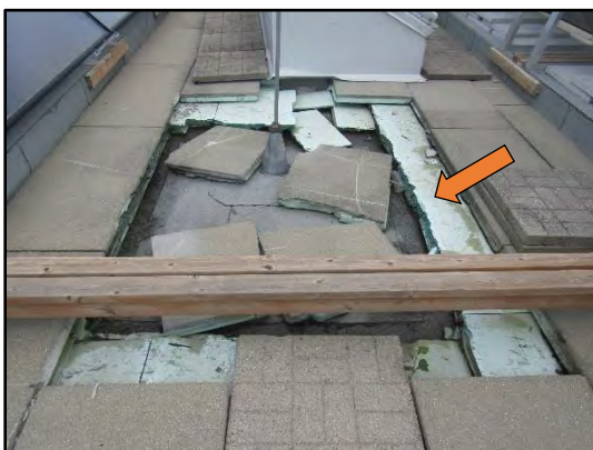
Damaged precast concrete pavers and insulation observed on the upper level roof area.
