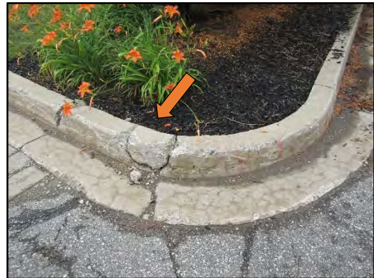
Deterioration in the concrete curb observed on the south portion of the site.
