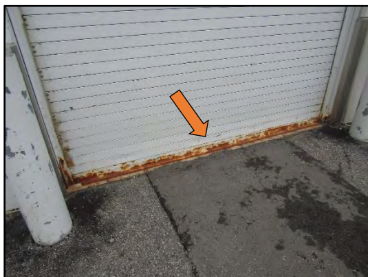
Corrosion on the steel roll-up door observed on the west elevation of the building.
