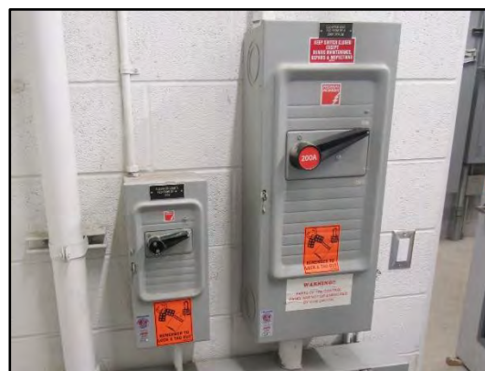
Various disconnect switches.
