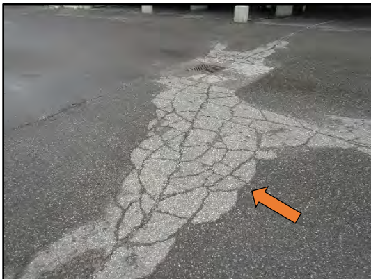
Cracking in the asphalt pavement observed on the west portion of the site.
