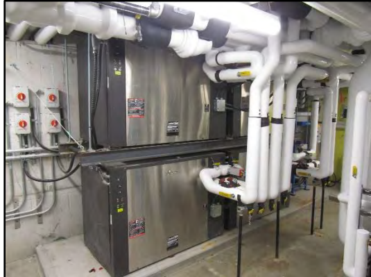
ClimateMaster water-to-water heat pumps.
