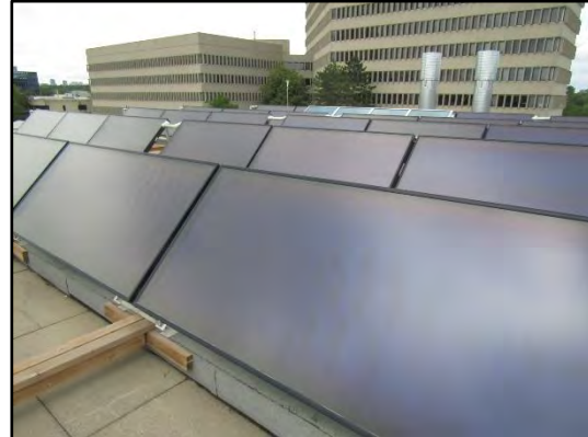
Hydronic solar thermal panels.
