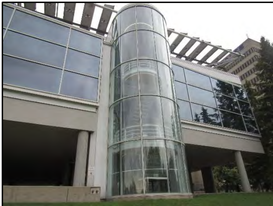
General view of the original curved curtain wall system on the east elevation of the building.
