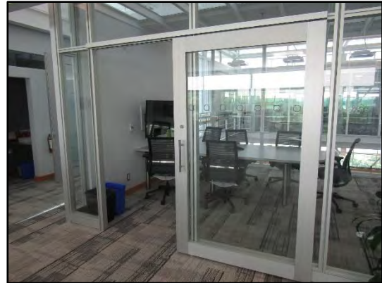
General view of a horizontal SG door with aluminum frame in the interior office space.
