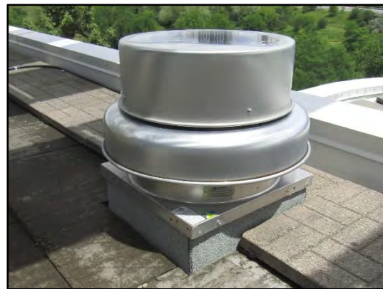
Greenheck main stairwell exhaust fan.
