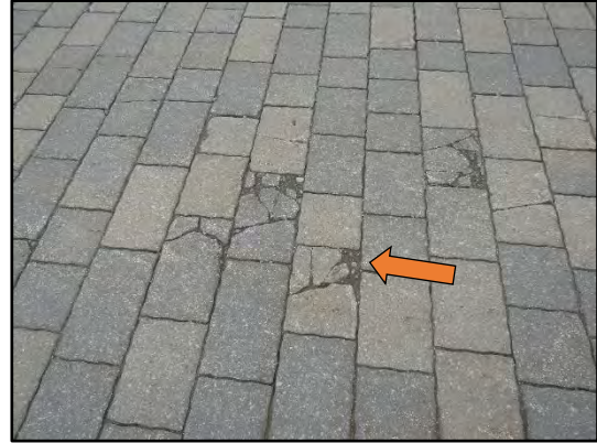
Cracking and deterioration in the pavers observed on the south portion of the site.
