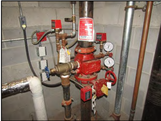
Sprinkler main riser and shut-valve.
