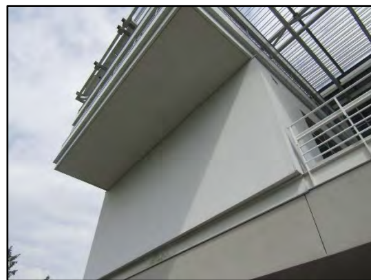
General view of the insulated vertical aluminum panels.
