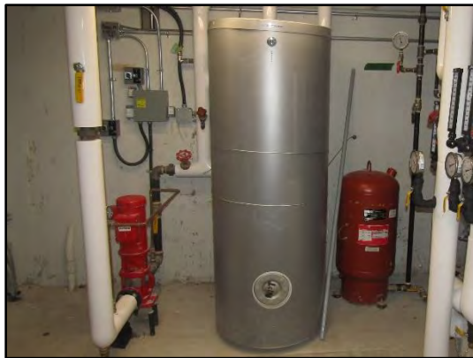
Indirect hot water tank heater and recirculation pump.
