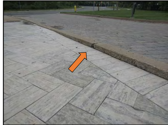
Settled and uneven stone pavers observed on the south portion of the site, which may pose a potential tripping hazard.
