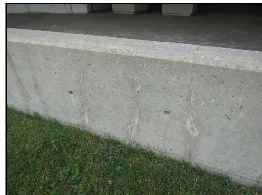
Minor cracking in the concrete retaining wall observed on the east portion of the site.
