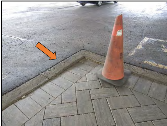
Settled and uneven stone pavers observed adjacent to the main entrance of the building, which may pose a potential tripping hazard.
