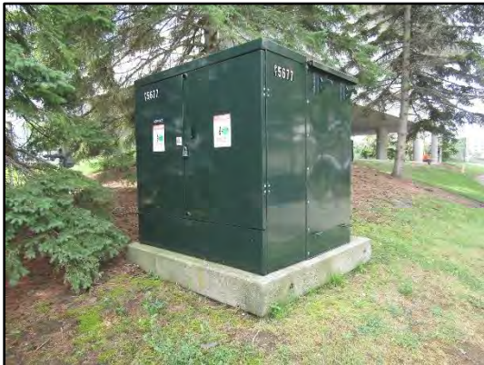
Main concrete pad-mounted municipal transformer.
