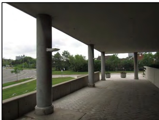
General view of the steel columns (covered with fibre cement panels).
