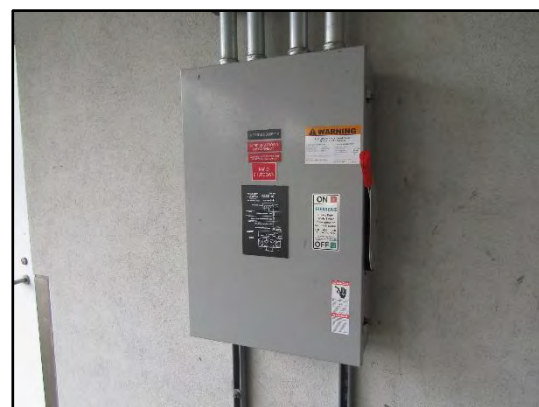
Solar photovoltaic energy system rapid shutdown disconnect switch.
