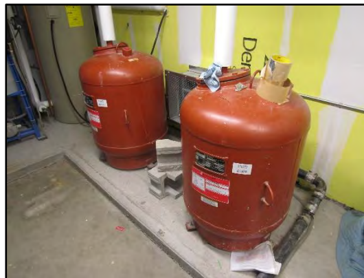
Bell & Gossett expansion tanks.
