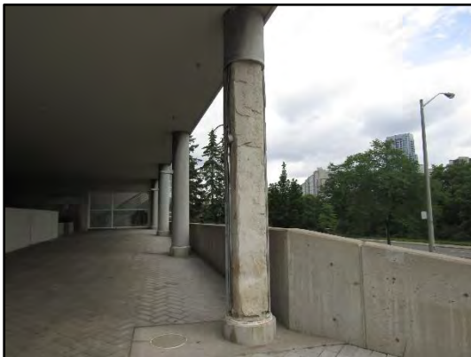
General view of the columns which are cladded with fibre cement panels. Note: Severely damaged fibre cement panels were observed on the southeast portion of the building.
