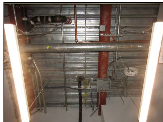
General view of a steel column supporting a composite floor slab (profiled steel deck overlain with concrete).
