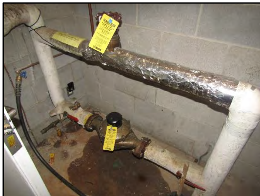
Main water incoming line and water meter.
