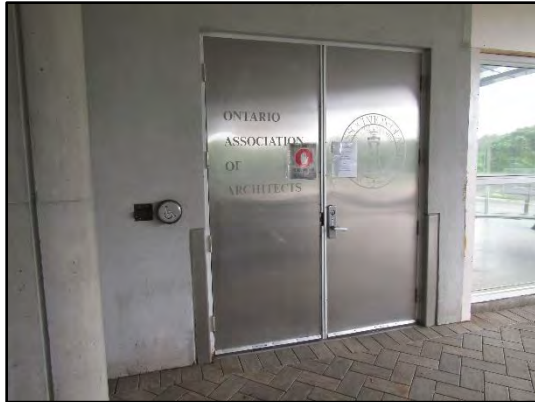
General view of the aluminum doors with metal frames at the main entrance.
