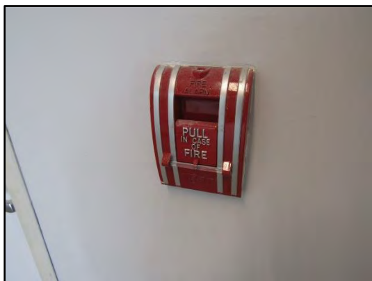
Typical manual pull station.
