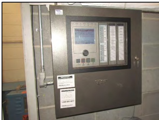
EST fire alarm main control panel.
