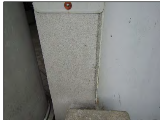
Cracking in the exterior wall joint sealant observed on the east elevation of the building.
