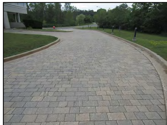
General view of interlocking stone pavers observed on the south portion of the site.
