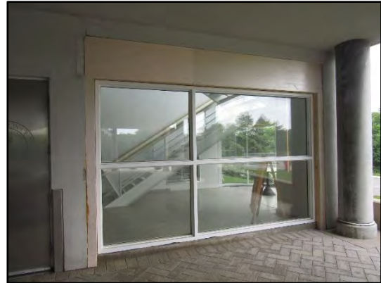
Unfinished EIFS observed at the main entrance on the ground level (scheduled to be refinished subsequent to the site visit).
