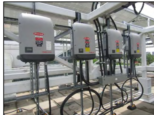
Fronius solar power inverters.
