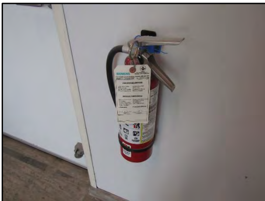
A typical dry chemical fire extinguisher.
