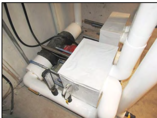
Plate and frame heat exchangers.
