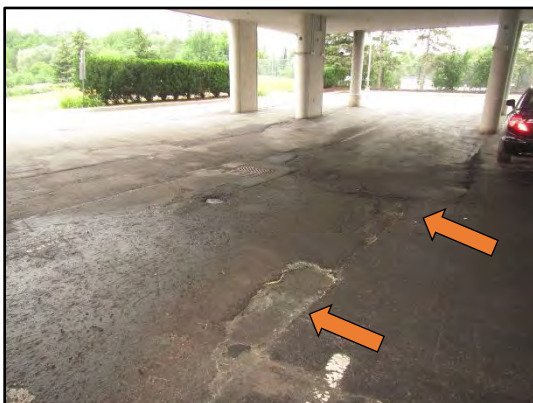
Deterioration in the asphalt pavement observed on the ground level.
