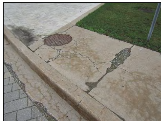
Cracking in the concrete walkway observed on the southeast portion of the site.
