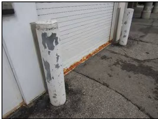
General view of the steel bollards filled with concrete. Note: Areas of peeling/flaking paint on the steel bollards were observed on the west elevation of the building.
