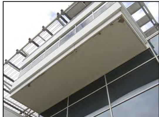
Flaking/peeling coating on the EIFS observed on the soffit on the south elevation of the building.
