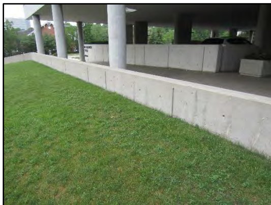
Cast-in-place concrete retaining wall observed on the east portion of the site.
