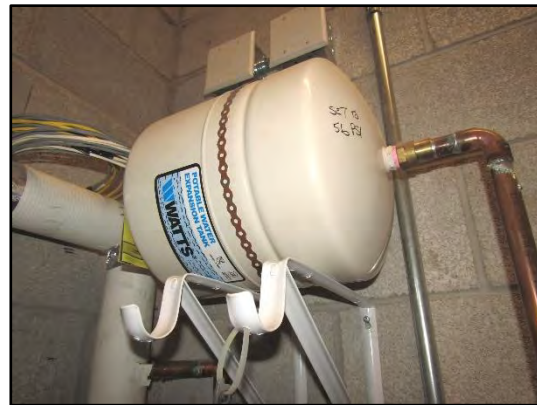
Potable water expansion tank.
