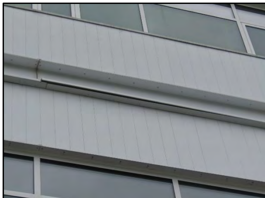
Detached aluminum panel observed on the west elevation of the building.
