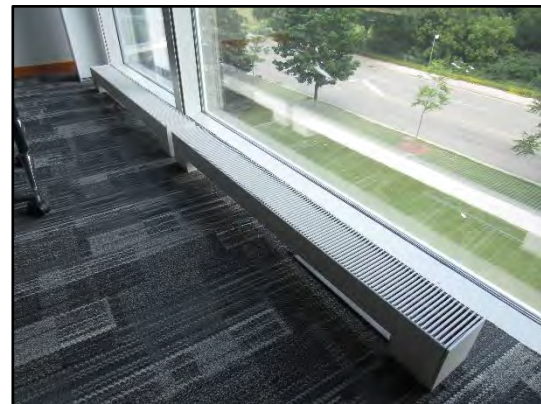
Floor mounted fan coils.
